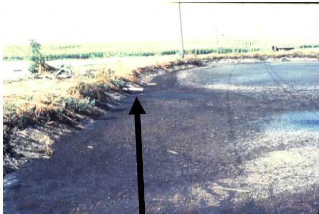
Operation Storage Lagoon
